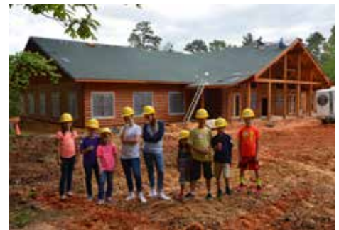
The Pines Catholic Camp new dining hall construction, April 2016.
