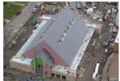
Construction is underway at the new Good Shepherd Catholic Church.
